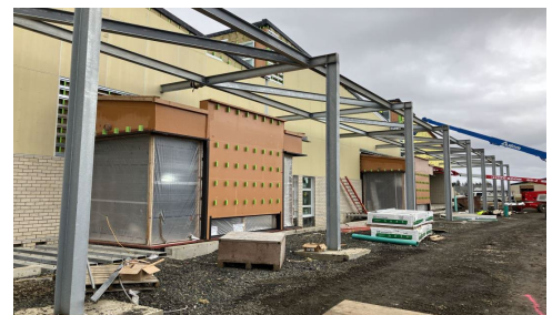
3 GHS Recreation Building, February 2023
